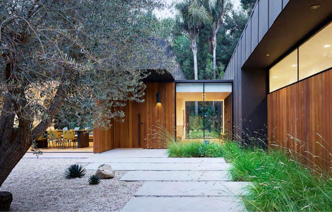
Laurel Canyon House - Exterior
